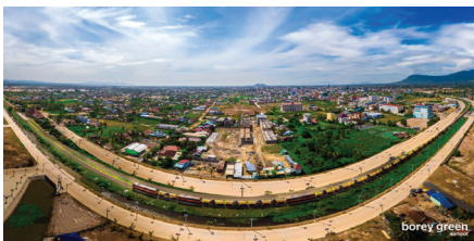
Train Station Road and Kampot Ring-Road
